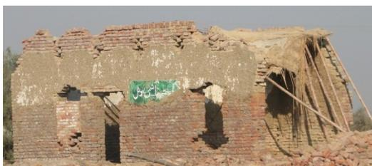
**Figure 4.11.** Damaged brick masonry building
