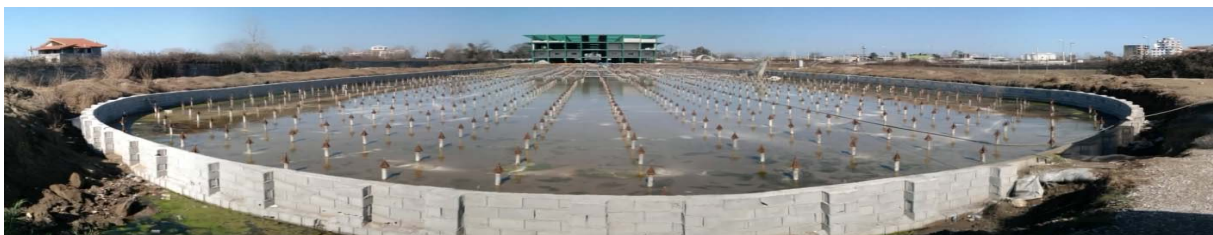
Figure 1.1. Micropiles can withstand axial and/or lateral loads, and may be considered a substitute for conventional piles.(Iran, MahmoodAbad, Narenjestan2- Southern site)
