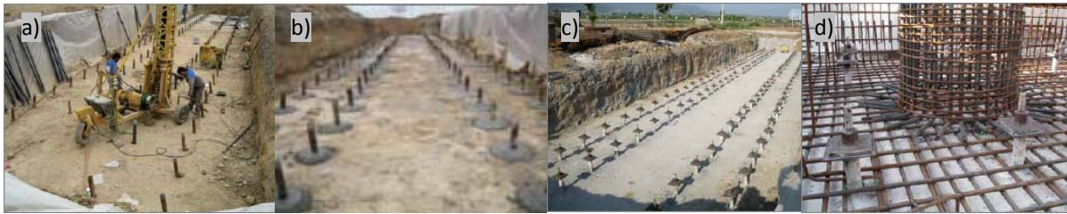
Figure 1.2. The recommended method for the micropile construction: a) driving a casing, b) fixing the casing and grouting, c) placing the reinforcement and d) installing the flange.
