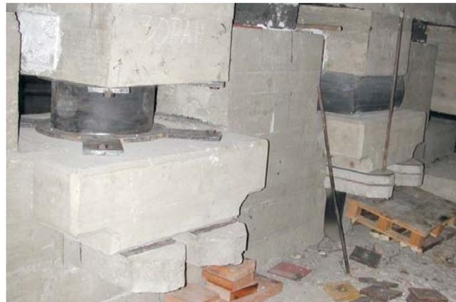
Figure. 1 Installed new and old bearing
