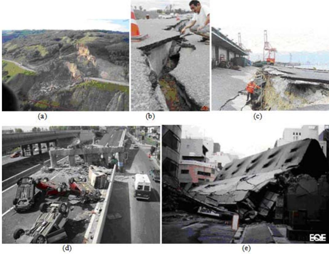
**Figure 2.** Various types of seismic hazards affecting roads serviceability: a) Landslide, b) Faulting, c) Liquefaction, d) Damaged bridges and e) Collapsed buildings
