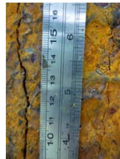
d) Cracks induced by corrosion damage
