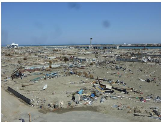
**Photo 2.** In Yuriage 4-chome near the fishing port, houses were totally lost, only foundations of wooden houses remain
