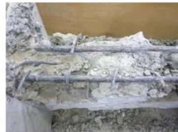
**Figure 16.** Stirrups with 90° hook**Figure 15.** Main reinforcement at beam ends
