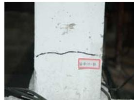
**Figure 11** Horizontal cracking at the bottom end of a column at 1st floor
