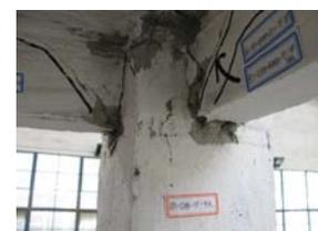
**Figure 16** Damage of the joint at 7th floor
