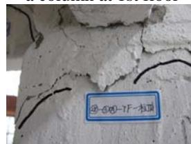
**Figure 15** Cracking at the top end of a column at 7th floor
