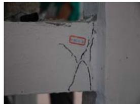
**Figure 10** Cross cracking at the end of a beam at 1st floor
