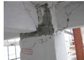
**Figure 12** Damage of the joint at 8th floor
