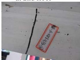
**Figure 13** Cracking at the end of a beam at 1st floor
