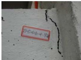
**Figure 9** Cracking at the end of a beam at 2nd floor
