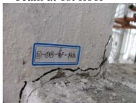
**Figure 14** Cracking at the bottom end of a column at 6th floor
