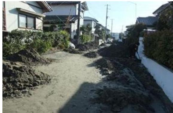
**Fig.2.3.** Many sand boiling in a residential section in Chiba
