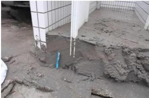
**Fig.2.2.** Sedimentation of the sand boiling in Urayasu
