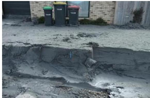
Fig.2.6. Sedimentation of the sand boiling in Christchurch (After Shock)
