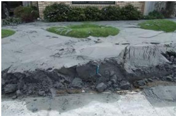
Fig.2.5. Sedimentation of the sand boiling in Christchurch (Main shock)
