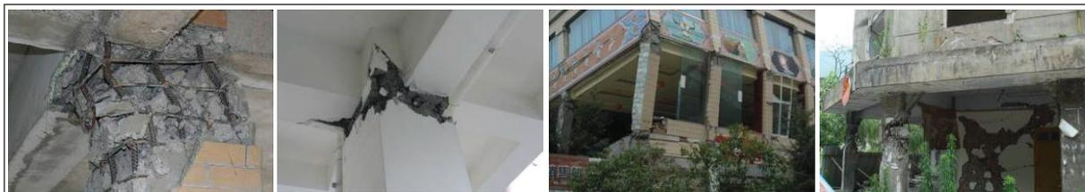
**Figure 1.1.** Damages of RC beam-column joint in the earthquake
