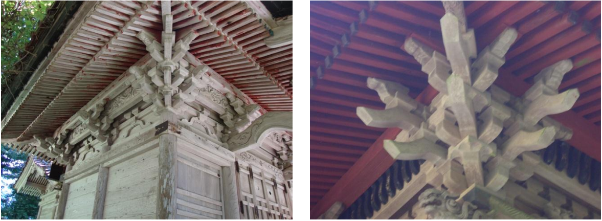
Figure 8. Detail of the entablature in the connection between column and roof
