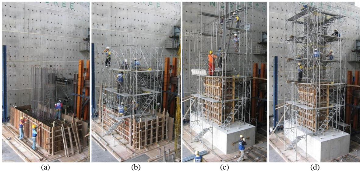
**Figure 3.** Construction photos for the conventionally detailed column (a) erection of the lower main bars; (b) binding of the reinforcing bars for the lower part; (c) erection and connection of the upper main bars; (d) binding of the reinforcing bars for the upper part
