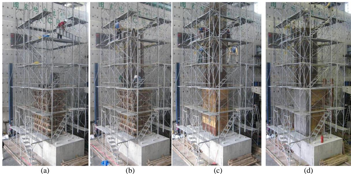
**Figure 2.** Construction photos for the proposed composite column (a) erection of scaffold (b) erection and connection of the steel section and part of the main bars; (c) installation of the pre-assembled hoop cage; (d) erection and connection of the remaining main bars.
