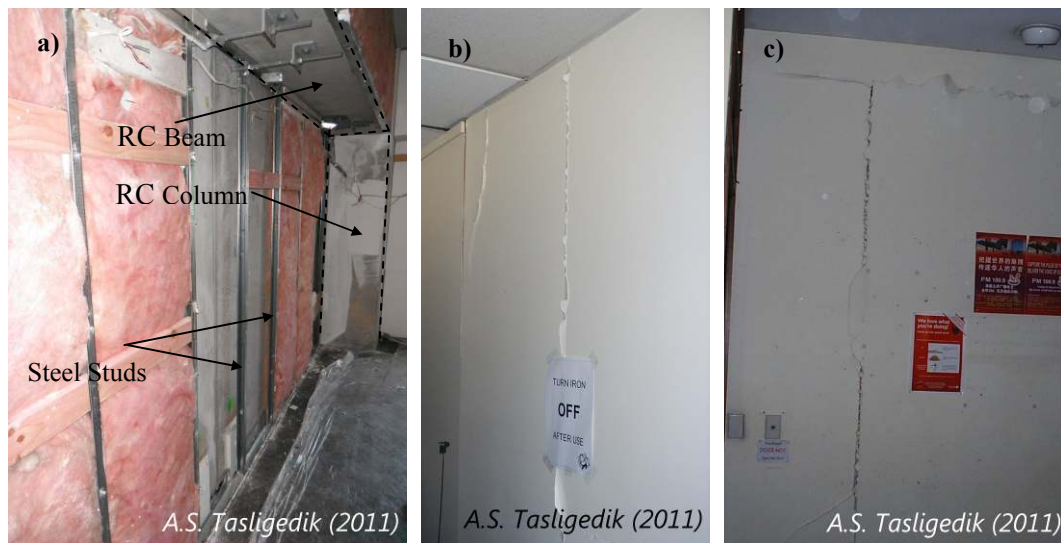
Figure 1. a) Drywall framing bounded by RC structural frame, b)-c) Observed damage at drywalls after February 2011 earthquake in Christchurch, New Zealand
