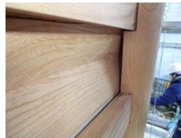
Fig.25 Crack of board wall.
