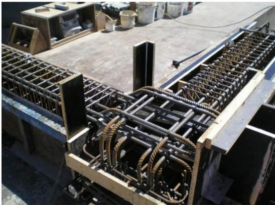
(a) Reinforcement cage in form prior to concrete pour.
