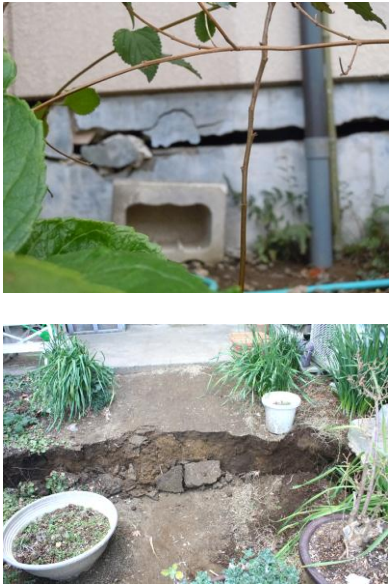
Figure 25. Deformation of Foundation soil and damage of foundation (point A)
