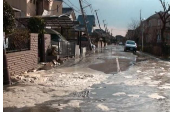
Figure 12 Sand spread over the road and inclined electric poles at Sodegaura district
