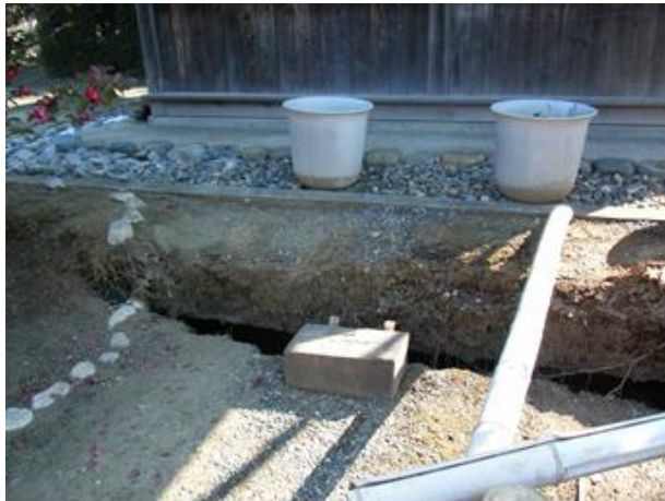
Figure 27. Subsidence of ground due to liquefaction at point B
