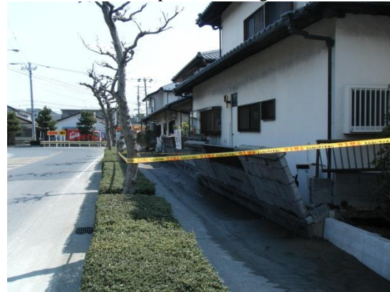
Figure 14. Sand spread and an inclined wall at Kasumi district
