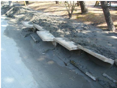
Figure 15. Damage of side ditch along the road at Sodegaura district.
