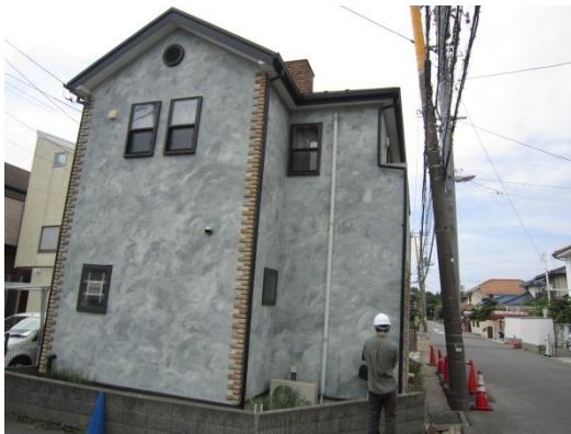
Figure 13. Settlement and inclination of a house at Kasumi district
