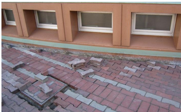
Figure 22. Subsidence of ground at M1 point
