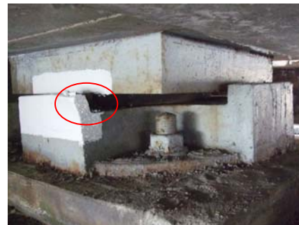
(a) Flexural Damage of Steel Bearing
