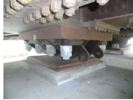
Photo5.2. healthy status of the LRB and Horizontal Bearing (Sendai area)
