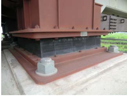
Photo5.2. healthy status of the LRB and Horizontal Bearing (Sendai area)
