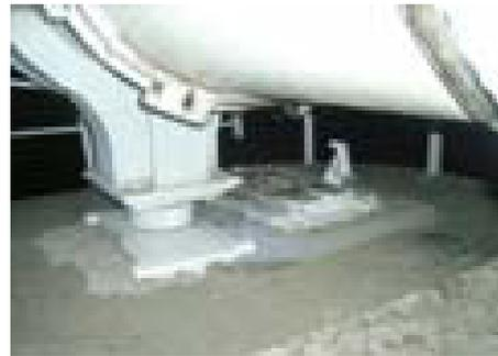
**Figure 2.4.** Damage of bearing at Pier 4
