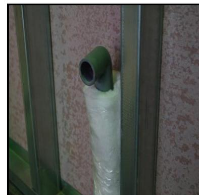
**Figure 6.** Water pipe wrapped by ceramic fiber carton
