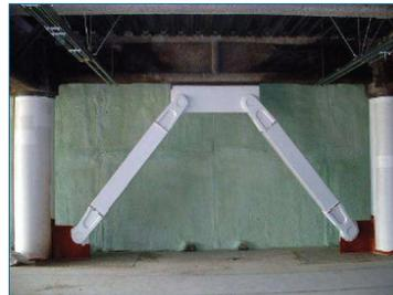
Viscous damping wall
