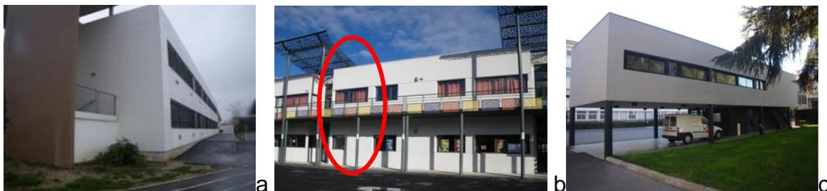
**Figure 2.1 :** parameter WA, examples of vertical bracing. a) bracing elements (shear walls) continuous on vertical, b) discontinuity between the 1st floor and the 2nd and c) soft story.
