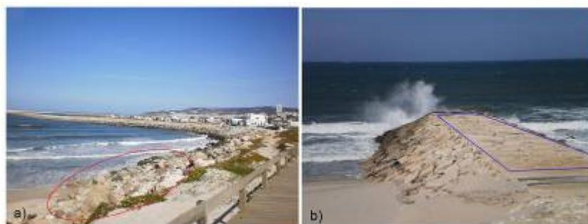
**Figure 4.3:** Photos taken during the field survey on April 2012: a) scattering of stone blocks of the south spur (shown in red) at Cabedelo; b) spur at Cova shows already some damage on its top, delimited by the blue line.
