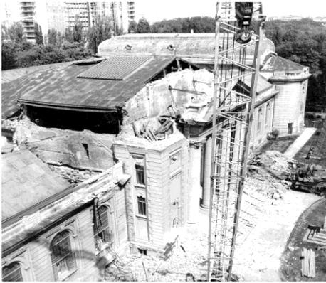
**Figure 3.1.a.** Faculty of Medicine, Bucharest. Seismic damage on March 4 1977 (Lungu et.al. 2000)
