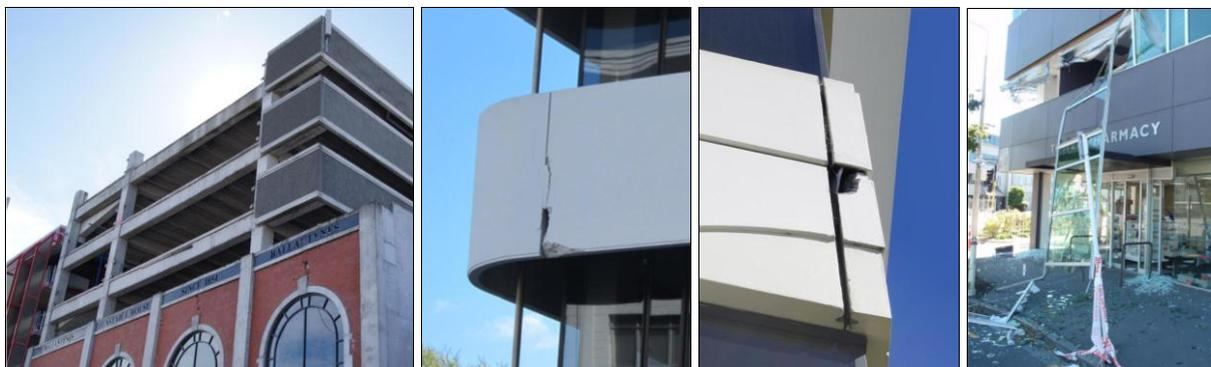
**Figure 1.1.** Cladding damage to multi-storey buildings in Christchurch CBD (Baird et al., 2012)
