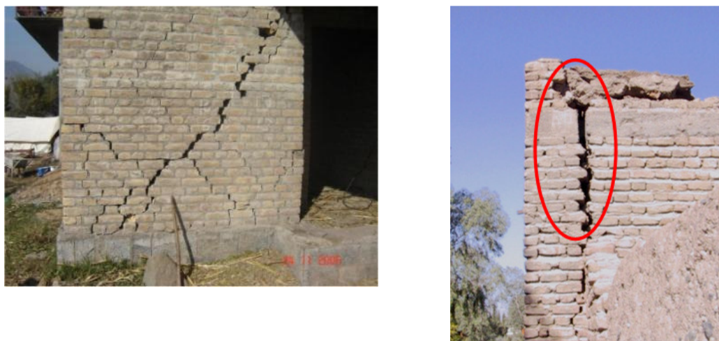
Fig 2.1 Diagonal shear failure, (left); Corner separation due to lack of integrity (right), 2005 Pakistan earthquake, Photo courtesy NSET
