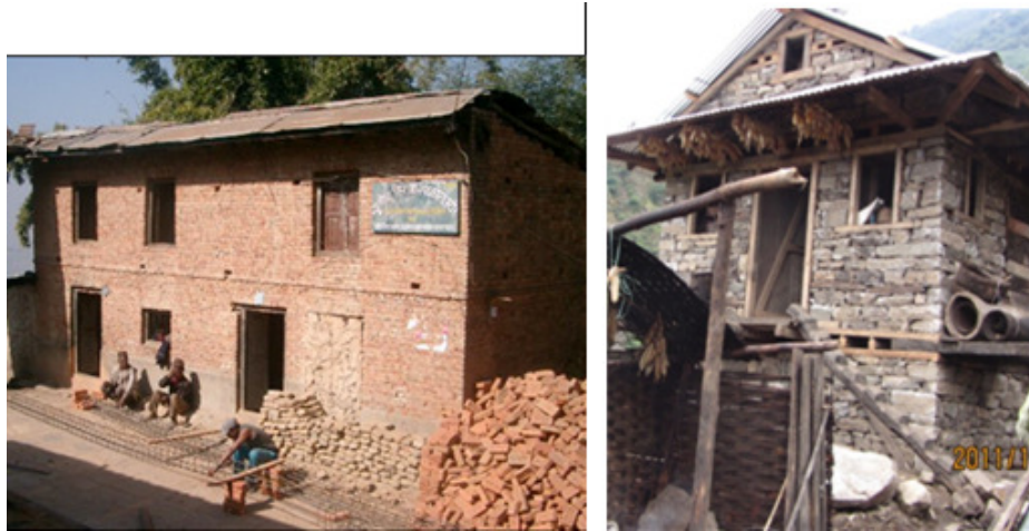
Fig 1.1 Typical brick (left) and stone (right) masonry buildings in Nepal
