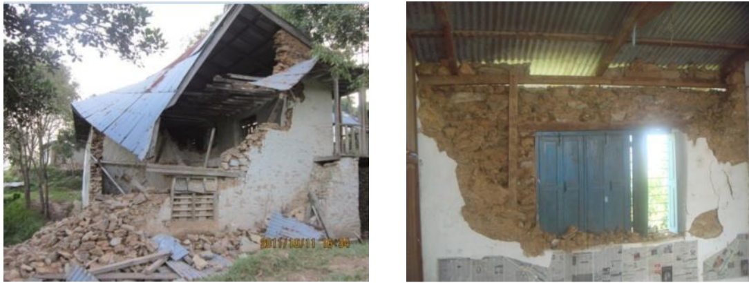
Fig 2.2 Failure of roof connection to wall (left); Collapse of inner wythe of stone wall due to lack of through stone (right), 18th Sept 2011 Taplejung Nepal earthquake, Photo courtesy NSET
