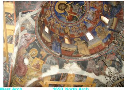
**Figure 8b.** Damage of the cruciform vaults and the pendentives supporting the central dome.
