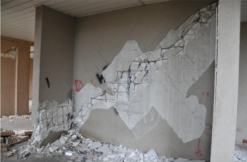
**Figure 1.3** Shear failure of the wall in an apartment building during the L’Aquila earthquake
