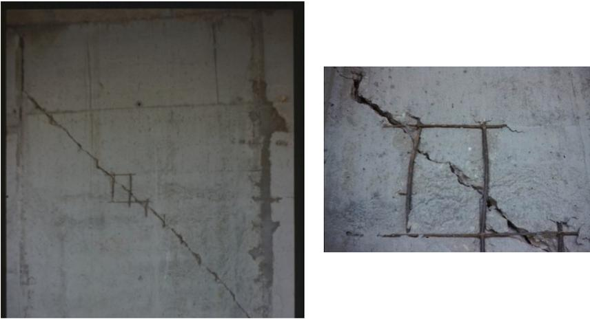
**Figure 1.2** A pier in a coupled wall damaged during the 1979 Montenegro earthquake
