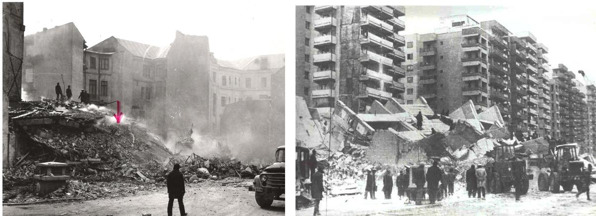
**Figure 2.** Full collapse and extreme loss of volume in 1977 in case of pre-1940 RC structure, Al. Sahia No. 1-3, (left) and collapse of pre-1977 OD 16 Block shear-wall section (right).
