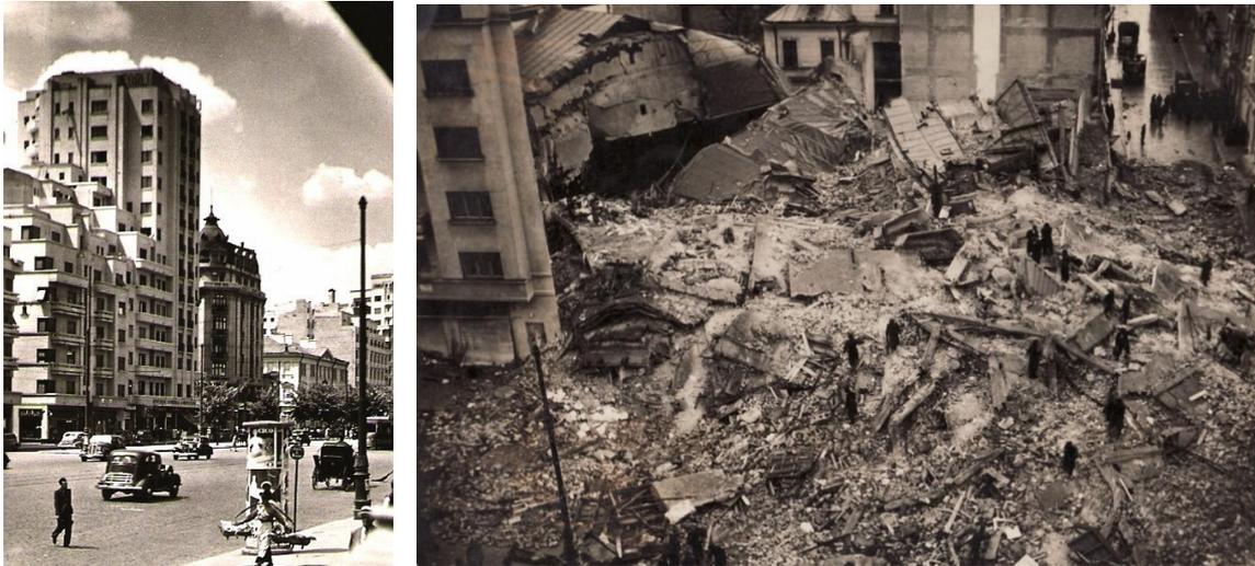
**Figure 1.** Carlton Block before collapse (left) and immediately after collapse (right)
