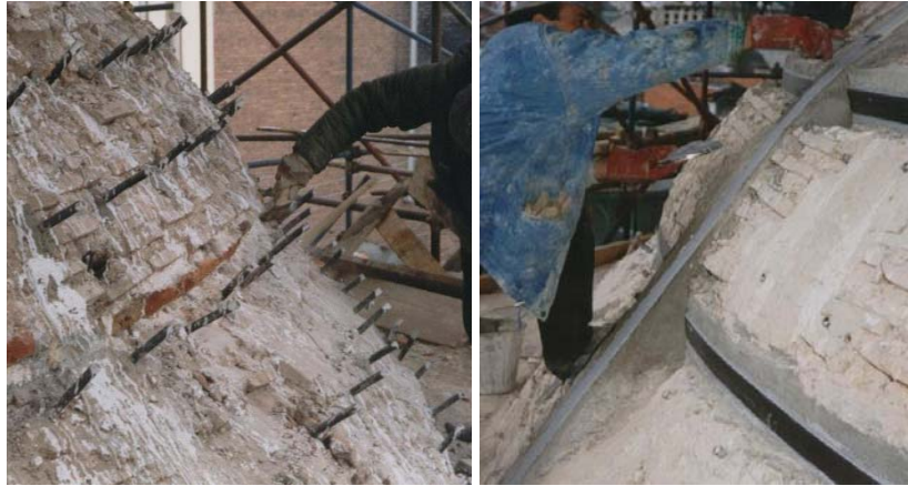
Figure 3. Injection of cracks and built in carbon strips.
