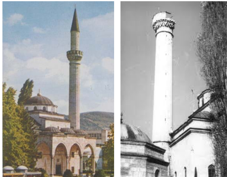
Figure 7. 1969 Earthquake damages on Ferhadija's minaret that cracked above balcony.
