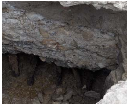
Figure 5. Detail of existing foundations with emphasis on oak micro-piles.
