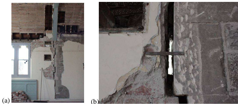
Figure 6. Interior views of Old Boy's High, showing interaction between adjacent buildings: (a) distant view, (b) close up view.
