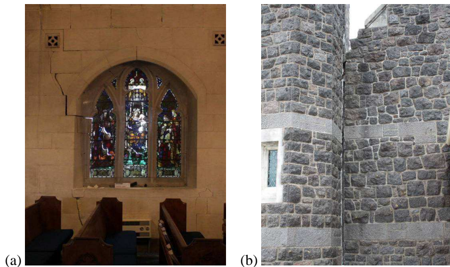
Figure 5. (a) St. Barnabas' Church, internal view. (b) St. Mary's Anglican Church: detachment of the bell tower from the nave
