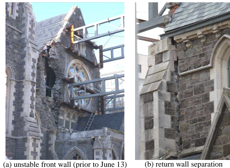
Figure 7. Christchurch Anglican Cathedral: out-of-plane overturning of the front façade
