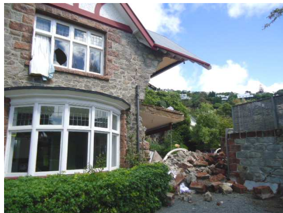
Figure 8. Rockvilla dwelling with complete collapse of the north and east façades
