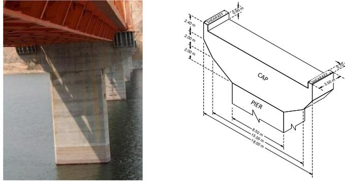
**Figure 6.** Reinforced Concrete Piers and Hammerhead cap of the Infiernillo II Bridge
