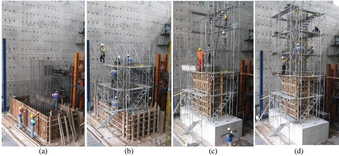
**Figure 3.** Construction photos for the conventionally detailed column (a) erection of the lower main bars; (b) binding of the reinforcing bars for the lower part; (c) erection and connection of the upper main bars; (d) binding of the reinforcing bars for the upper part
