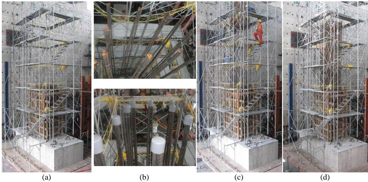
**Figure 2.** Construction photos for the proposed multi-spiral stirrup column (a) erection of scaffold (b) the capping of three vertical bars together with a cover; (c) installation of the pre-assembled multi-spiral stirrup cage; (d) fix position of the multi-spiral stirrup cage.
