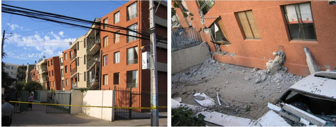
**Figure 3.** Damage of Don Tristán building after the 2010 Chile earthquake: (left) general view from the southwest, and (right) the first floor level resting directly on the ground at the basement level (the remains of totally crushed columns can be observed)
