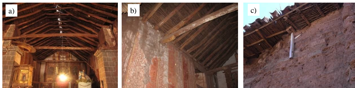
Figure 4. Roof's structure and structural details: a) nave's trussed roof; b) wooden tie-beams; and c) timber anchors
