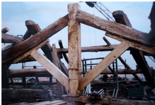
Figure 4. The truss after the intervention has acquired a king post scheme.
