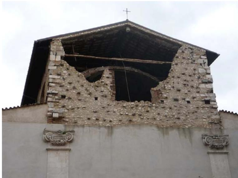
Figure 1. Façade of the church of S. Biagio Amiterno, L'Aquila, with the tympanum collapsed after the earthquake of 2009
