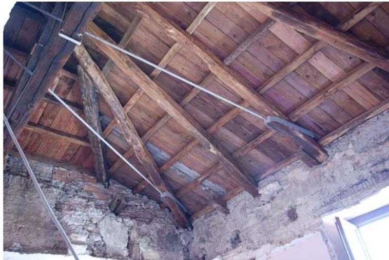
Fig. 5. Low-mass intervention on a timber roof in L'Aquila.
