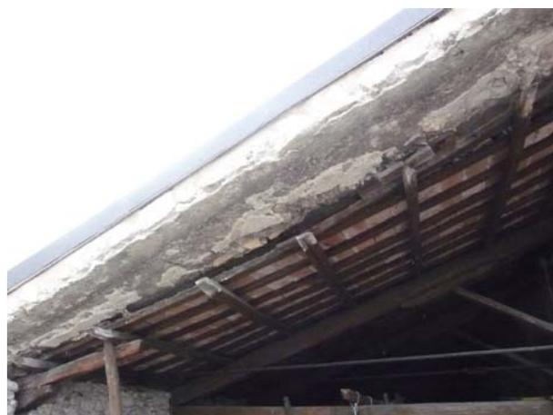
Figure 2. The roof structure loaded with a brick slab bordered with a concrete ring beam.
