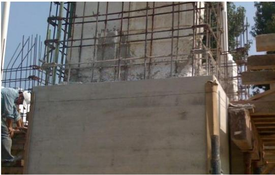
c) Concrete shear walls.
