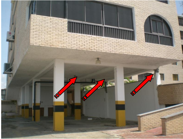
Figure 2. View of damage in short column. West Unit (A. Urich)
