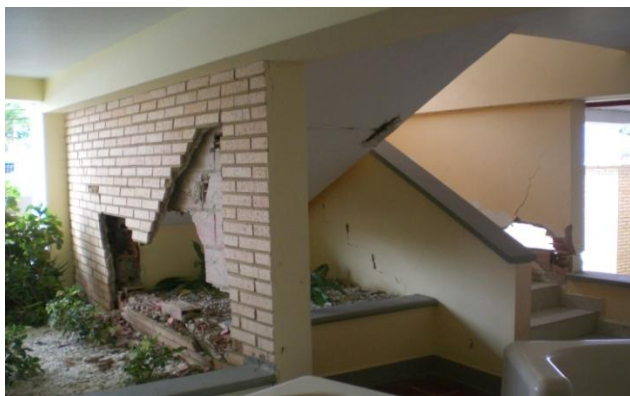
Figure 6. Damage in East staircase in the ground floor in the North Unit
