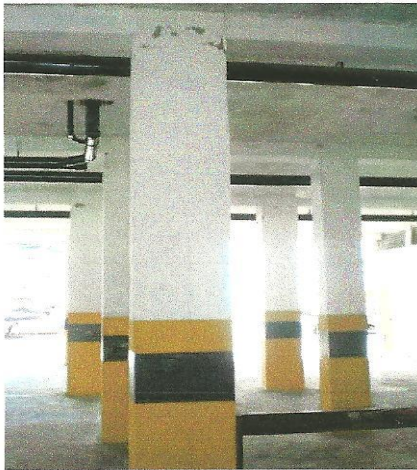
Figure 4. Cracking and crushing of concrete on top of the column (plastic hinge) in East Unit (A. Urich)
