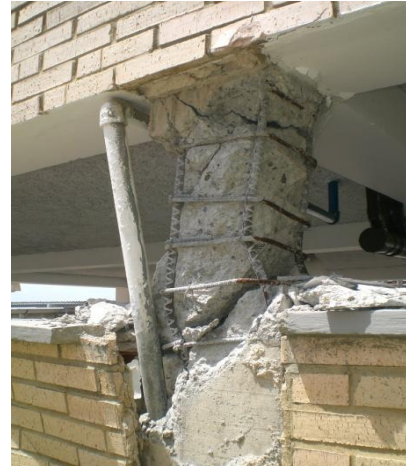
Figure 3. Detail of damage in short column of Figure 2 (A. Urich)
