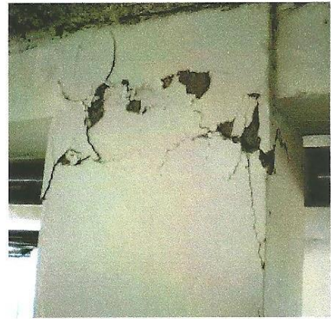
Figure 5. Detail of cracks at the top of the column of Figure 4 (A. Urich)
