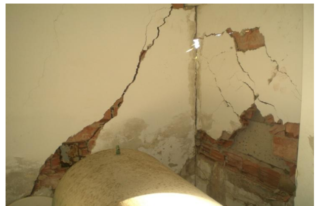
Figure 5. Detail of cracks at the top of the column of Figure 4 (A. Urich)
