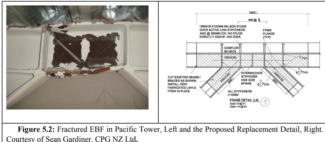
**Figure 5.2:** Fractured EBF in Pacific Tower, Left and the Proposed Replacement Detail, Right. Courtesy of Sean Gardiner, CPG NZ Ltd.
