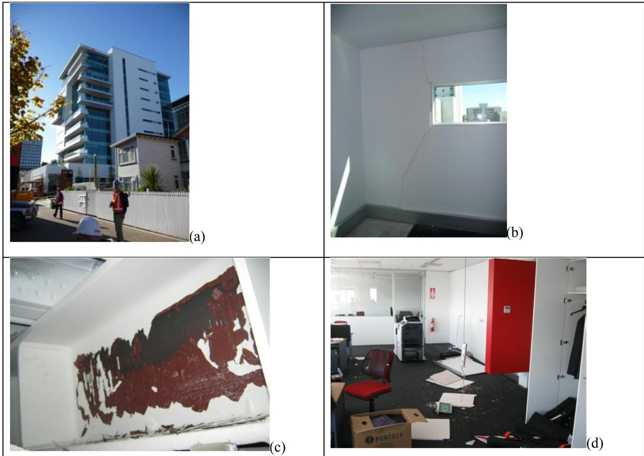
**Figure 3.1** Club Tower [Photos by M. Bruneau and C Clifton]: (a) Global view; (b) cracking of partition in cantilevering portion of story; (c) paint flaking of EBF link in the ceiling space; (d) general view of office showing minor disruption
