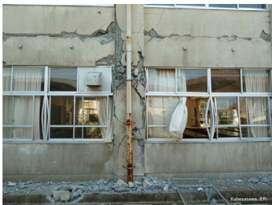
(c) Damages to column in north frame
