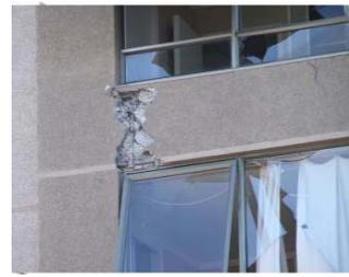
**Figure 1.2.** Photo for failure of coupling beam in 2/27/2010 Chile Magnitude 8.8 earthquake
