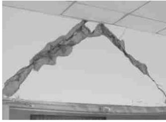
**Figure 1.1.** Photo for failure of coupling beam in 5/12/ 2008 wenchuan earthquake, China
