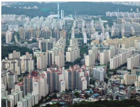
Figure 1.1. Photo of RC residential buildings in Korea
