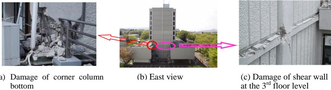
Photo 2. Damage feature of bottom of one of the damaged four corner columns at 3<sup>rd</sup> floor of THU building
