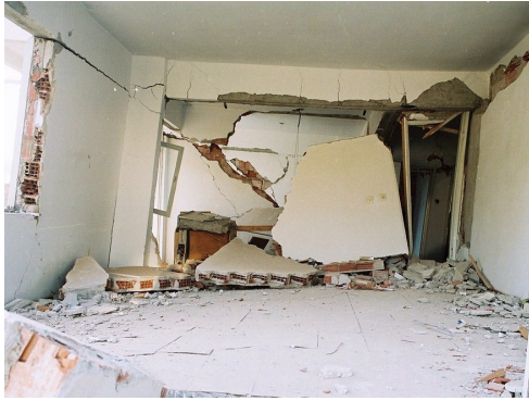
Figure 1. Collapse of infill-brick wall to out of plane Figure 2. Pancake crush of RC frames with infill-brick wall
