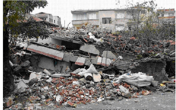
Figure 1. Collapse of infill-brick wall to out of plane Figure 2. Pancake crush of RC frames with infill-brick wall
