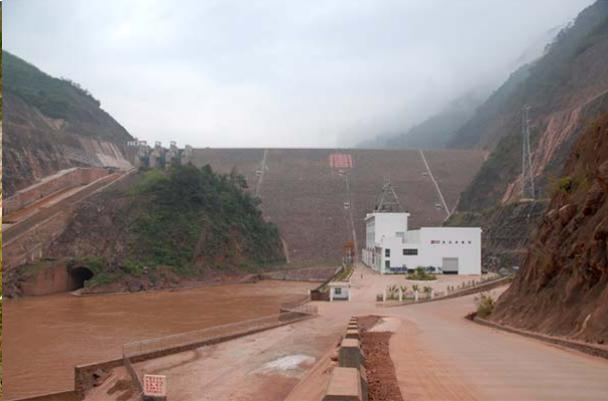
Figure 4. Longma concrete face dam
