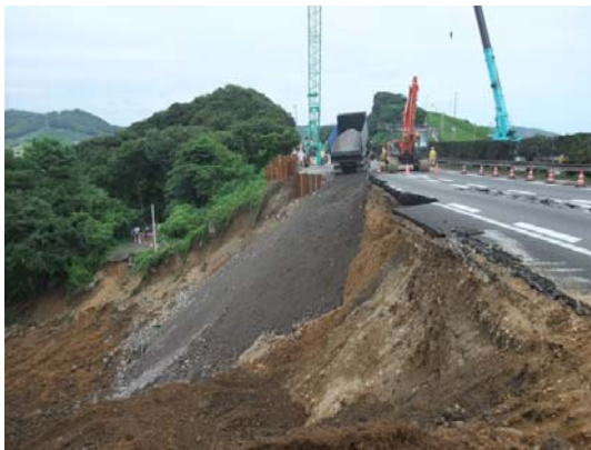
Figure 2. Failed slope of Tomei Expressway at Makinohara
