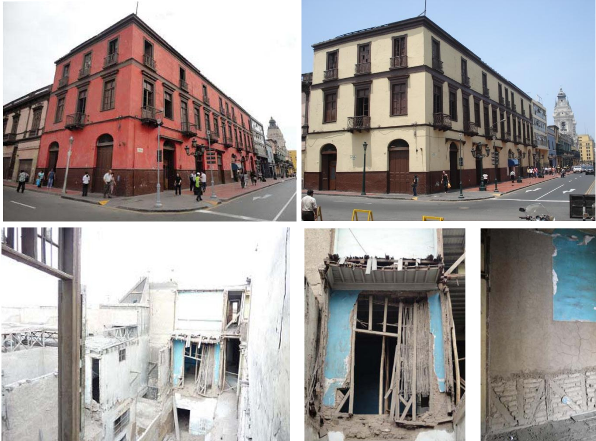
Figure 2. Typical adobe-quincha construction and structural condition details
