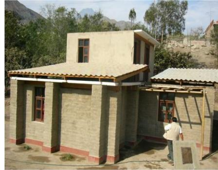
**Figure 3.** Construction of model seismic house of adobe
