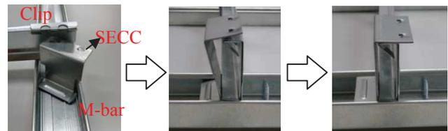
1. SECC is inserted in M-bar and set 2. The clip covered by SECC 3. Reinforcement completion
