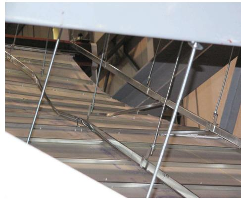
(a) Clip dropout process before falling of the M-bar (c) Failed situations of the ceiling elements
