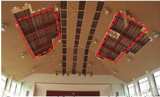
(a) Damage to metal furring suspended ceiling during the 2001 Geiyo Earthquake
