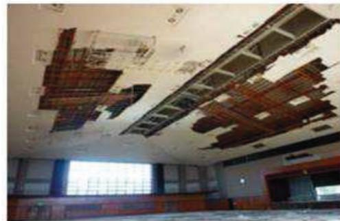
(b) Damage to metal suspended ceiling during the 2011 Great East Japan Earthquake
