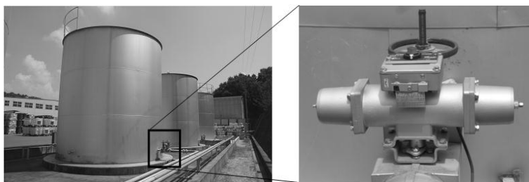
Photo 4.2. Example of shutdown system to close valves attached to a tank of toxic materials by EEW emergent alarm system developed by DPREC.
