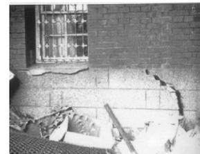
**Figure 9.** Wall body is bent (Chang, J. S. et al., 2001)
